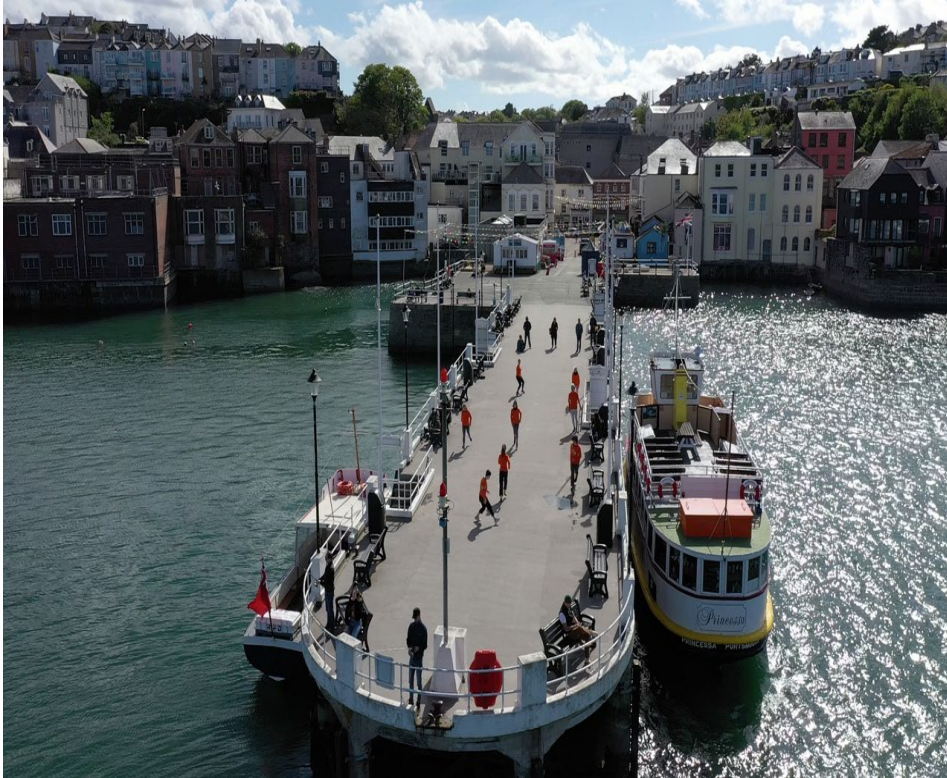
Figure 120, dAnCing LiNes , (2019/20), Prince of Wales Pier, Pillars and Beam
