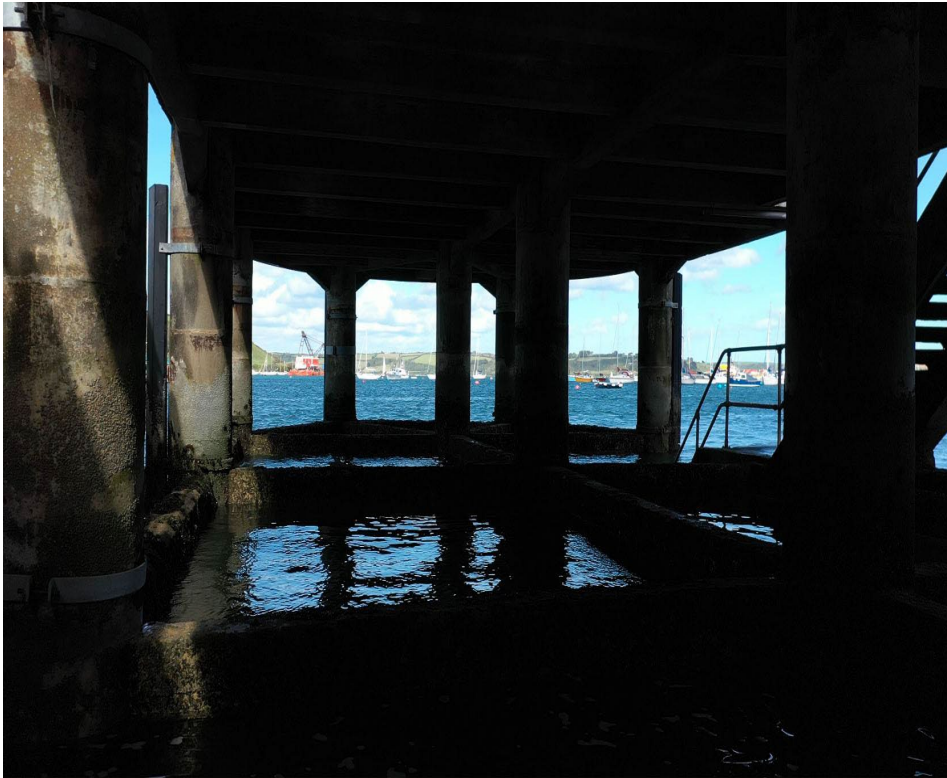
Figure 119, dAnCing LiNes , (2019/20), Prince of Wales Pier, Pillars and Beam
