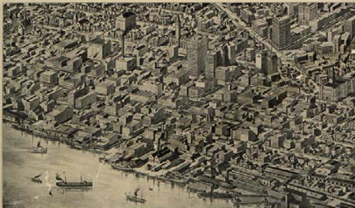
DETROIT 1900—SAME AREA AS VIEW ABOVE
